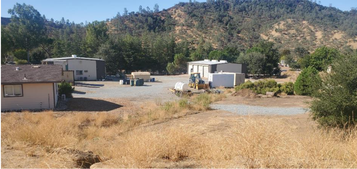
Photograph 1. Photograph of the existing wastewater treatment plant, facing southwest. October 6, 2022.
