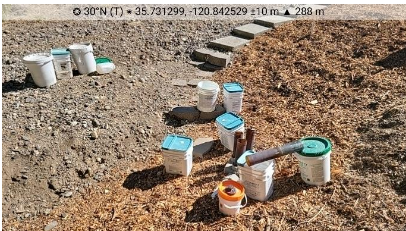
Photograph 3. Existing Dechlorination Facilities at Spray Field.
