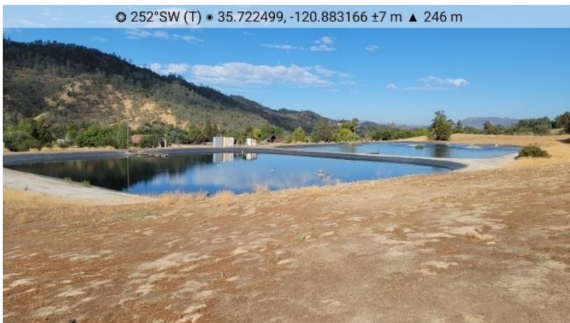
Photograph 1. Existing HRCSD Wastewater Treatment Ponds, Facing Southwest.
