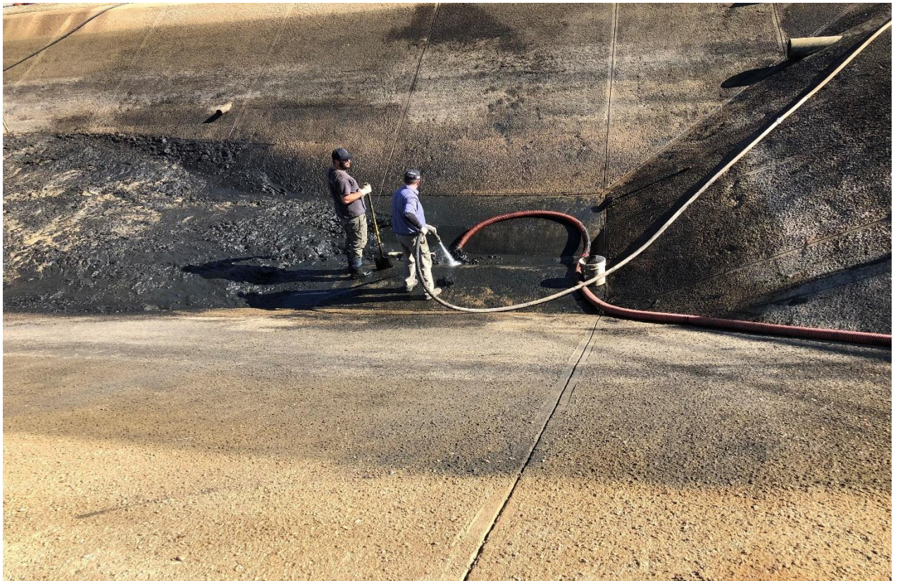
BACK WASH RECOVERY BASIN SLUDGE REMOVAL PROCESS
