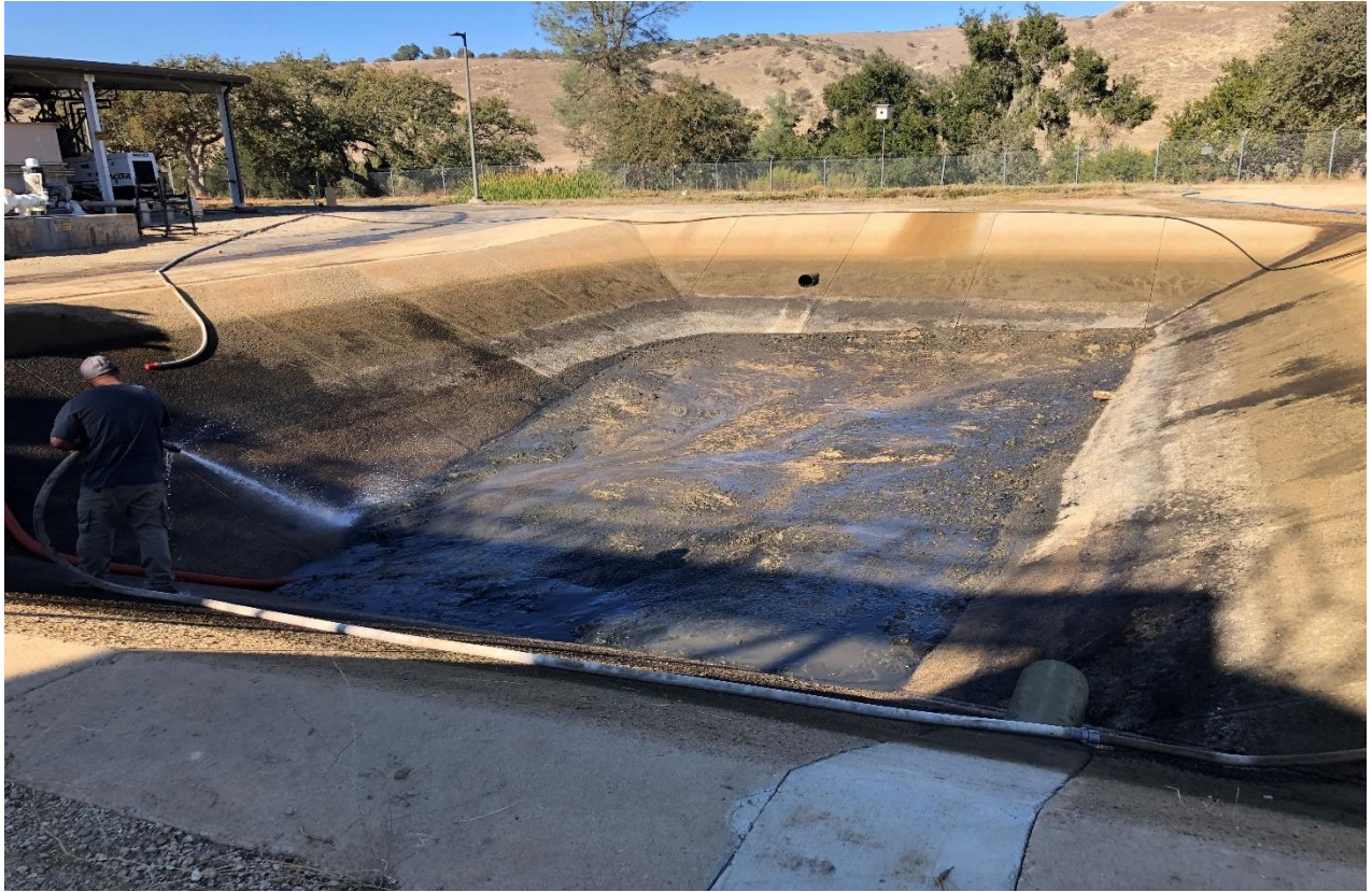
BACK WASH RECOVERY BASIN SLUDGE REMOVAL PROCESS
