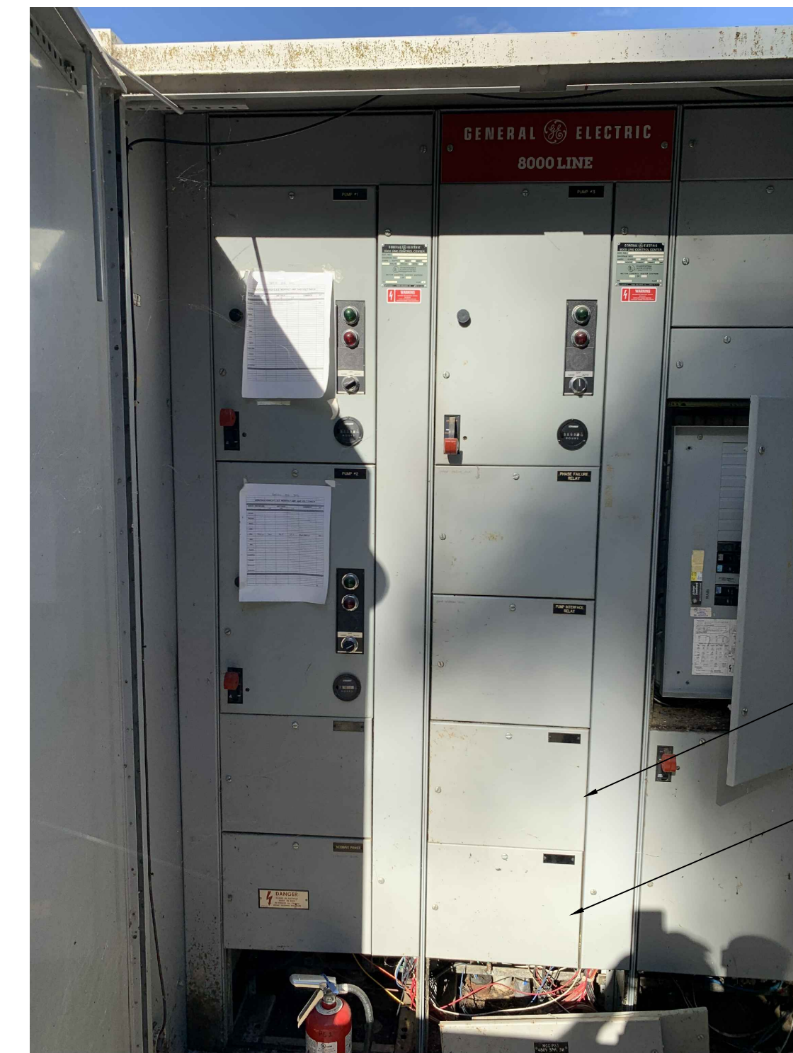
2 EXISTING MCC 'MSB' - PARTIAL INTERIOR NTS
