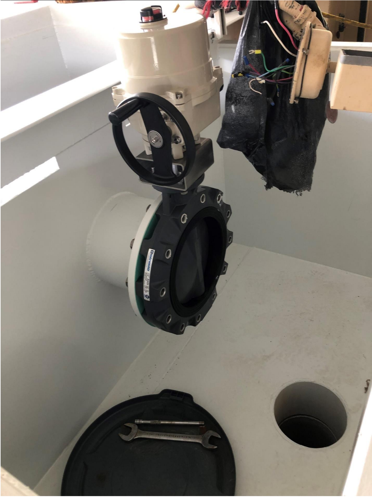
New Valve and Actuator at Filter Waste Location
