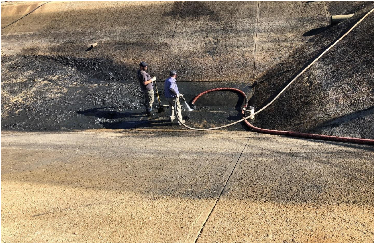
BACK WASH RECOVERY BASIN SLUDGE REMOVAL PROCESS
