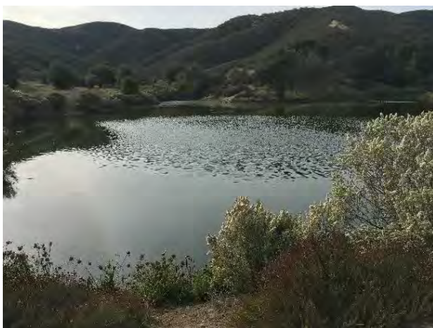
Figure 7 Pond 3 Effluent Storage Pond
