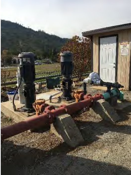
Figure 5 Existing Effluent Pump Station
