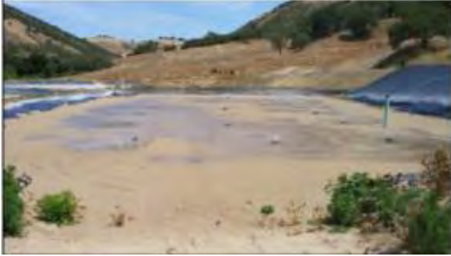
Figure 8 Existing Sand Filters
