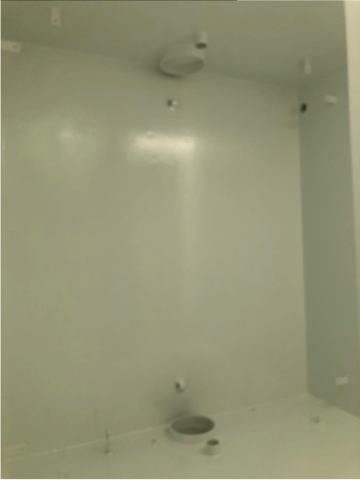
Filter #3 Painted - Looking at the Bottom of Polishing Side
