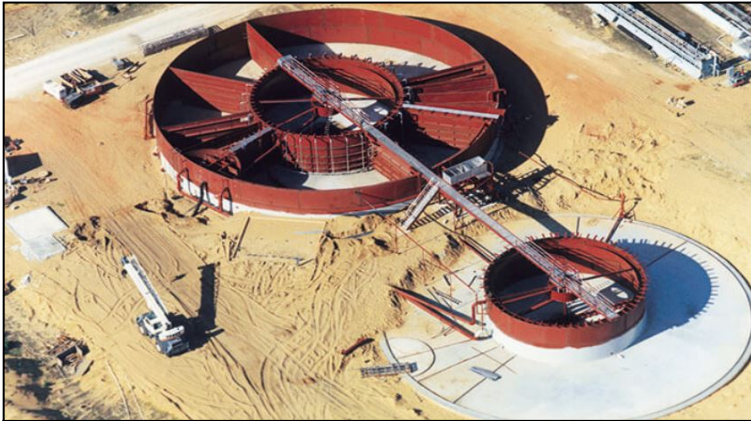
Figure 4-1: Evoqua Package Activated Sludge WWTP
